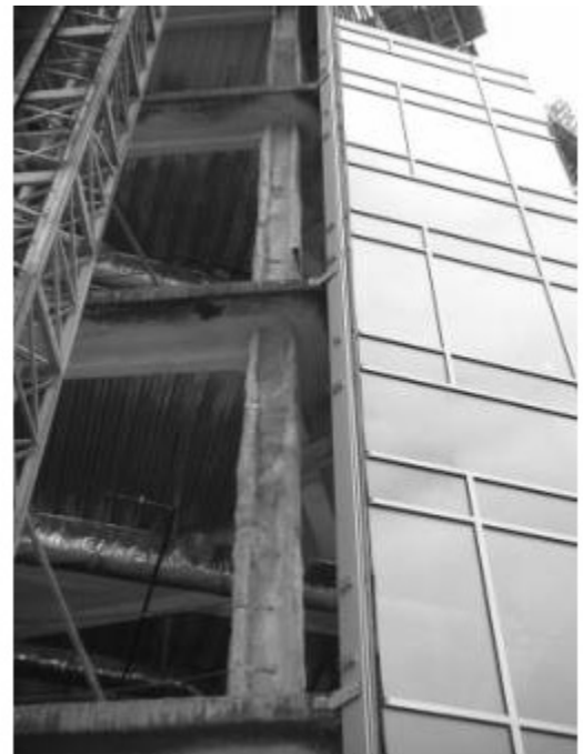
Fig. 2. Curtainwall in construction
