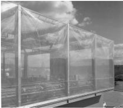
Figs. 10, 11. Waterworks Pavilion, Doncaster, England Use of ETFE as an exterior envelope material [Robinson-Gayle]
